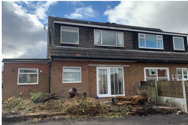
Photo 4: Rear of no. 5
