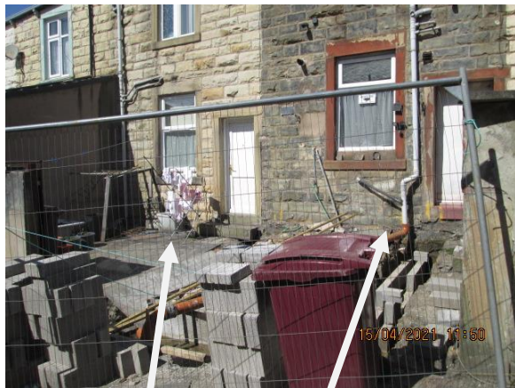
rear of 85 and 87 Brougham Street
