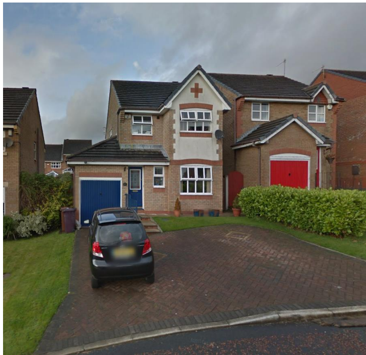
Photo 1: front of no. 50
