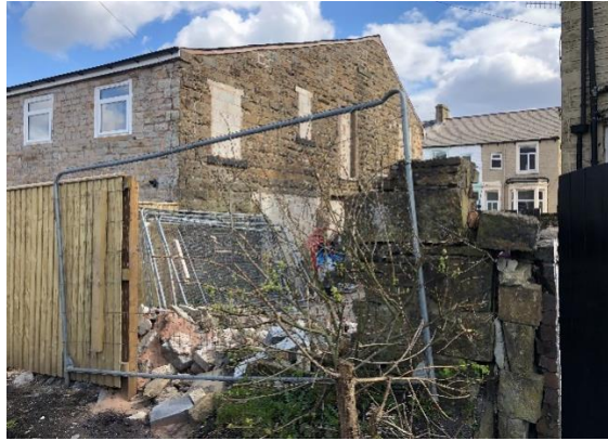
View across the site from the rear
