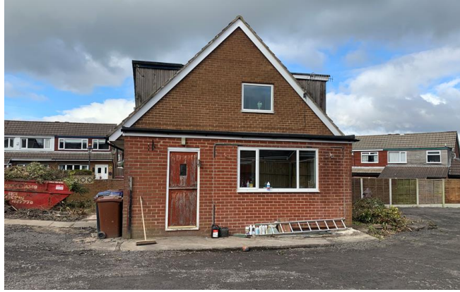
Photo 3: Side of no. 5
